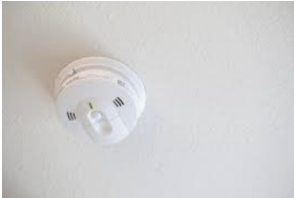
Mains-powered smoke alarm, ceiling-mounted, test button P-W5HJ44 · 2026-06-06 11:40
