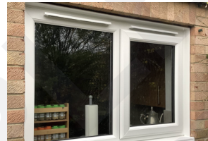
UPVC windows with trickle vents (background ventilation) P-VY1A61 · 2026-06-06 11:52
